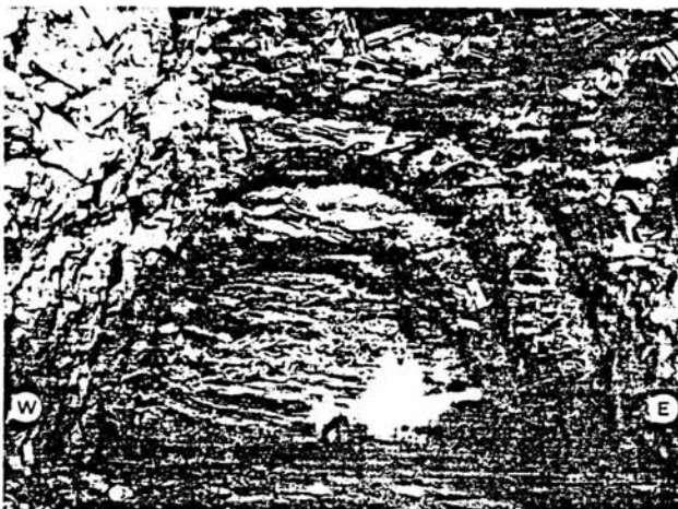
Fig. 3 Advance face (rock schistosity is readily apparent)
