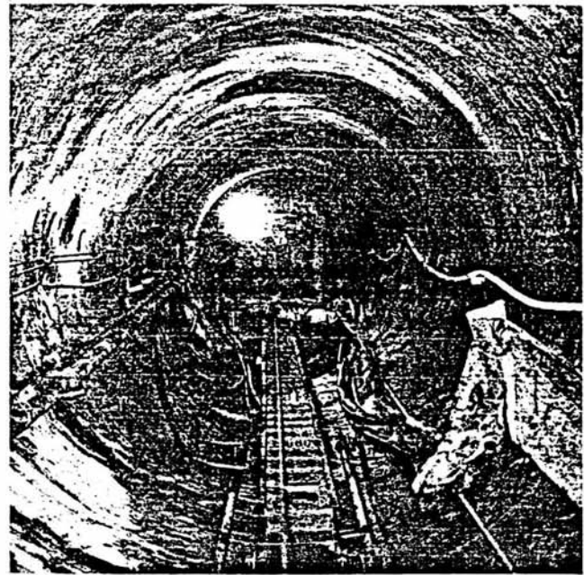
Fig. 7 First ventilation shaft bored
