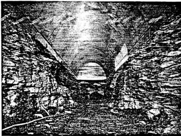
Fig. 6 Ventilation station room with side walls under construction
