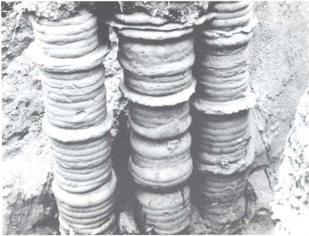
Fig. 5. Soil columns obtained by jet-grouting treatment
