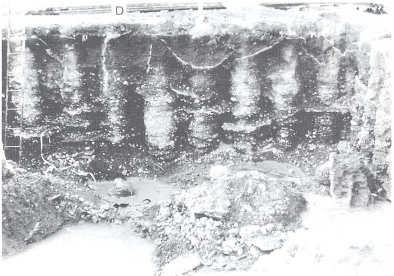
Fig. 6. Soil columns obtained by jet-grouting treatment
