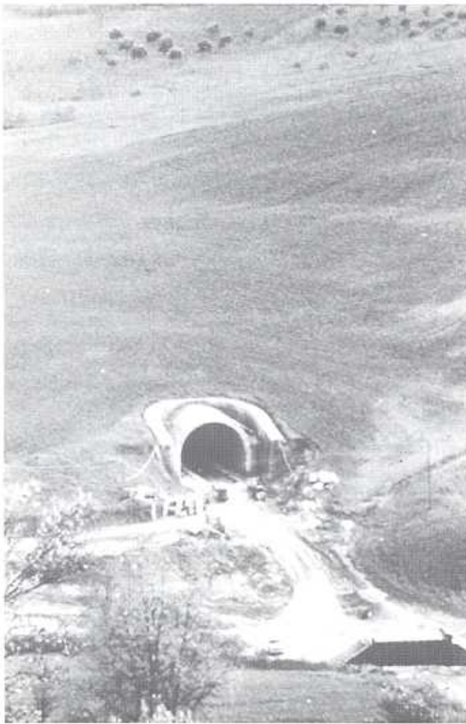
Fig. 20. Jet-grouting portal shell structure
