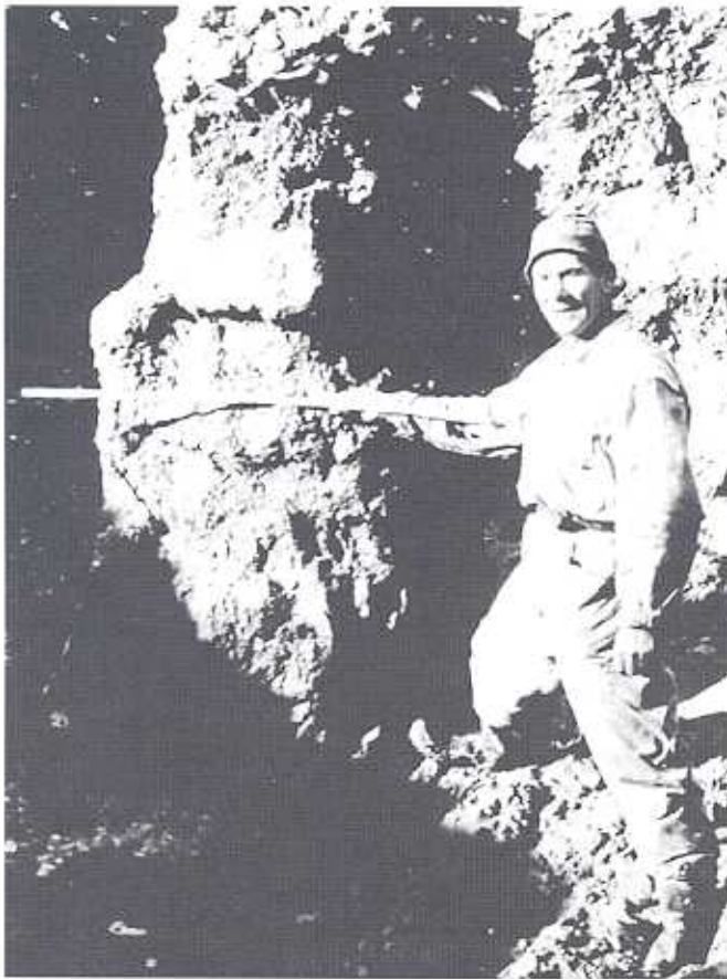
Fig. 7. Results obtained from jet-grouting treatment in stratified soil
