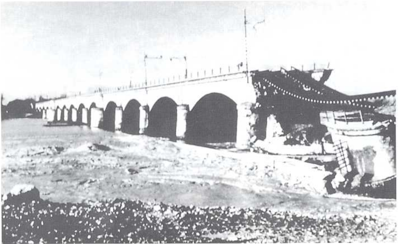
Fig. 30. Railway bridge over the Taro River (Italy) that collapsed due to the exceptional flooding in November 1982
