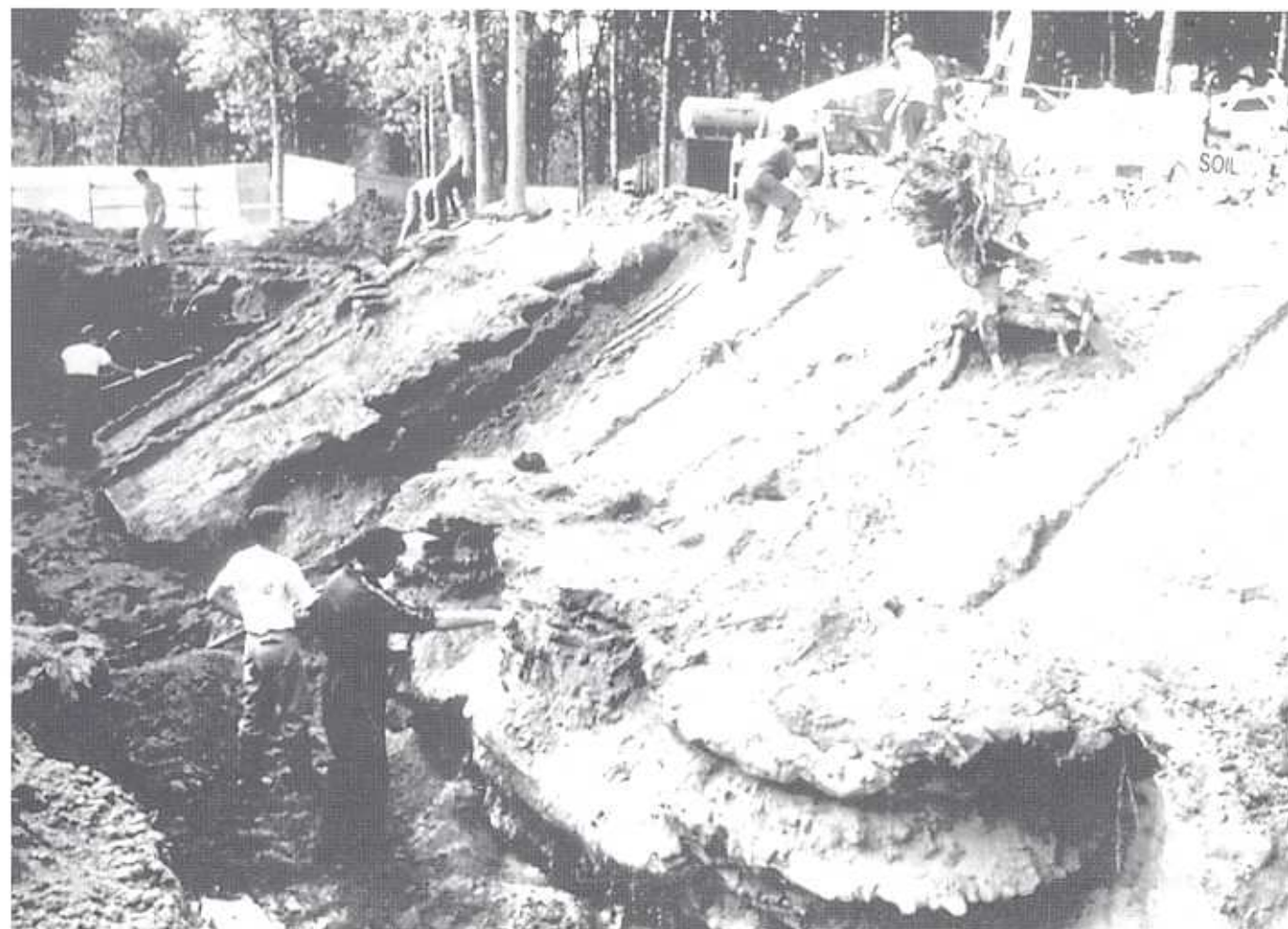
Fig. 15. Diaphragms of improved ground by jet-grouting
