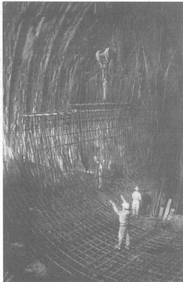
Figure 9. "Raticosa" tunnel: Steel reinforcement placing of invert
