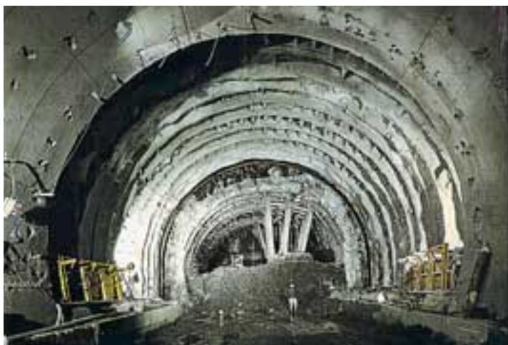
Photo 1: S. Stefano Tunnel (Italy, Genoa To Ventimiglia Rail Line, ground: tectonised and laminated marly-limestone flysch, overburden: 150 m, tunnel diameter: 12 m.). Collapse of the cavity.
