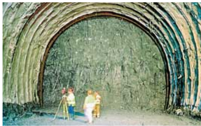
Photo 5: Pianoro Tunnel (Italy, Bologna to Florence High Speed Rail Line, ground: cemented silty sand, overburden: 150 m, tunnel diameter: 13.30 m.). View of the face reinforced with fibre-glass structural elements.
