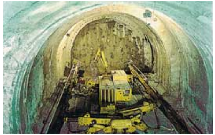
Photo 3: Vasto Tunnel: reinforcing of the advance core with fibre-glass tubes during full face excavation (according to A.DE.CO.-RS principles).
