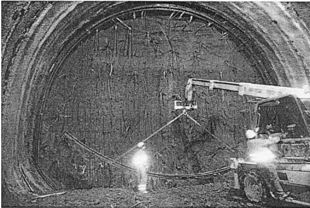
Figure 17 : The full-face excavation
