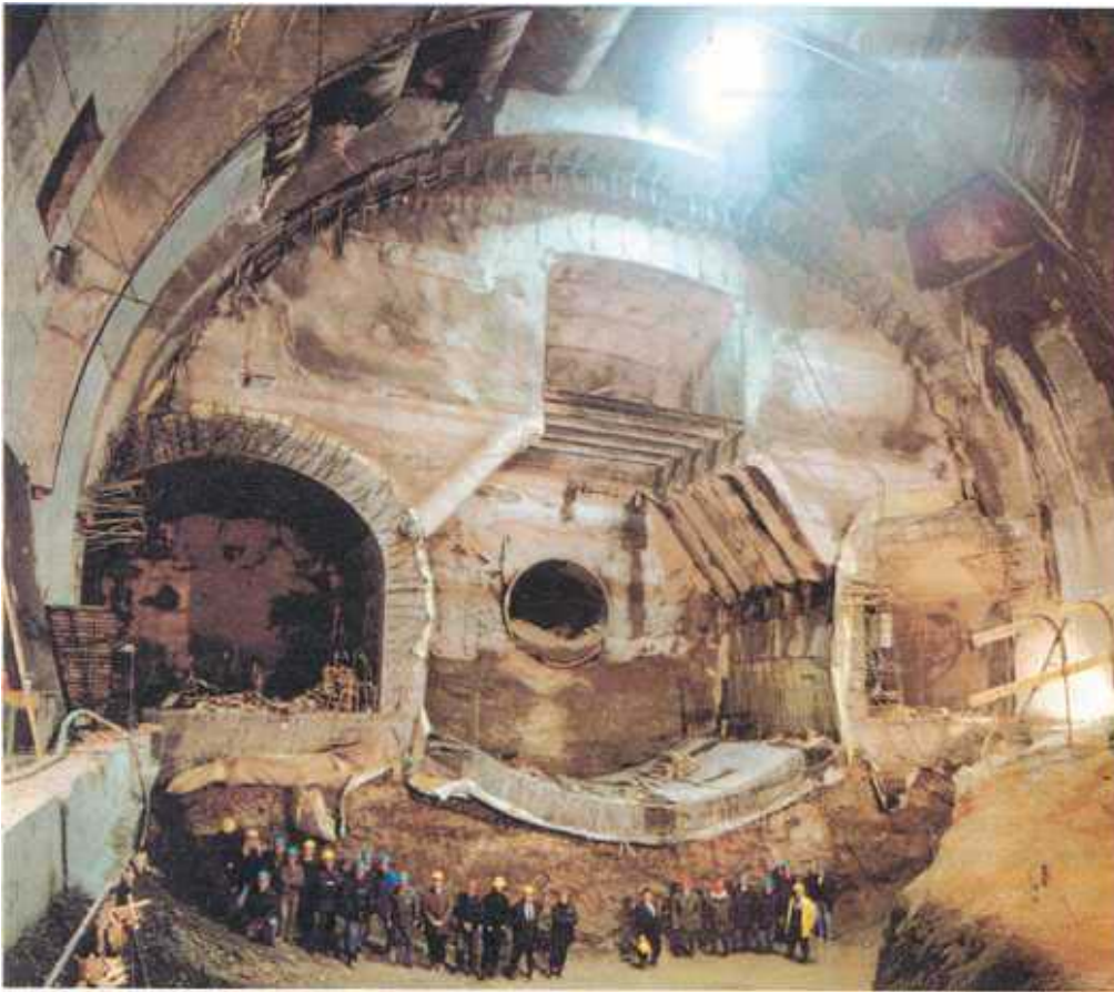
Venezia Station during construction
