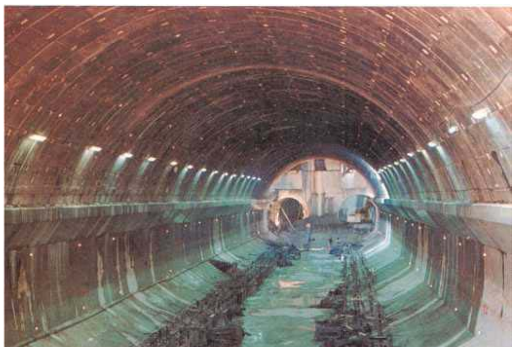
Baldo degli Ubaldi Station during construction of the tunnel invert
