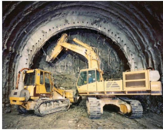
Fig. 20 Ancona to Bari rail line, Vasto tunnel: excavation stage.
