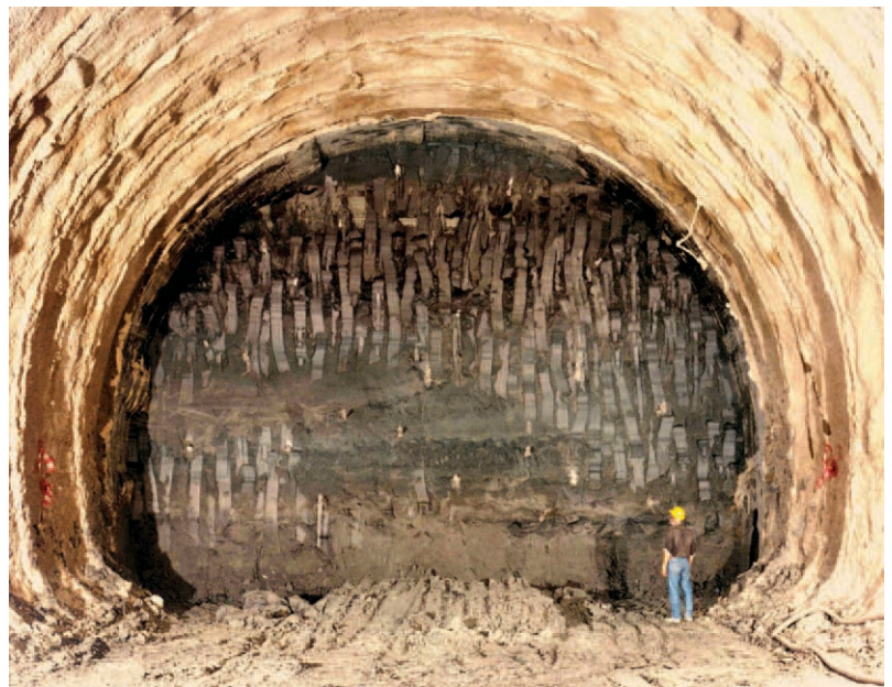
Fig. 8 Florence-Arezzo High Speed Rail Line, Terranova Le Ville Tunnel: view of the face reinforced with fibre-glass structural elements.
