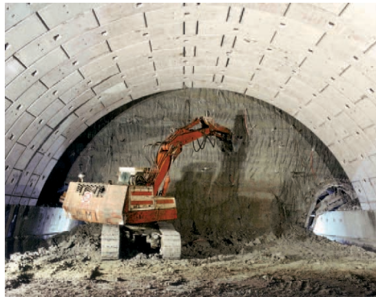
Fig. 21 Rome Metro: Baldo degli Ubaldi station: view of the face during the excavation stage.
