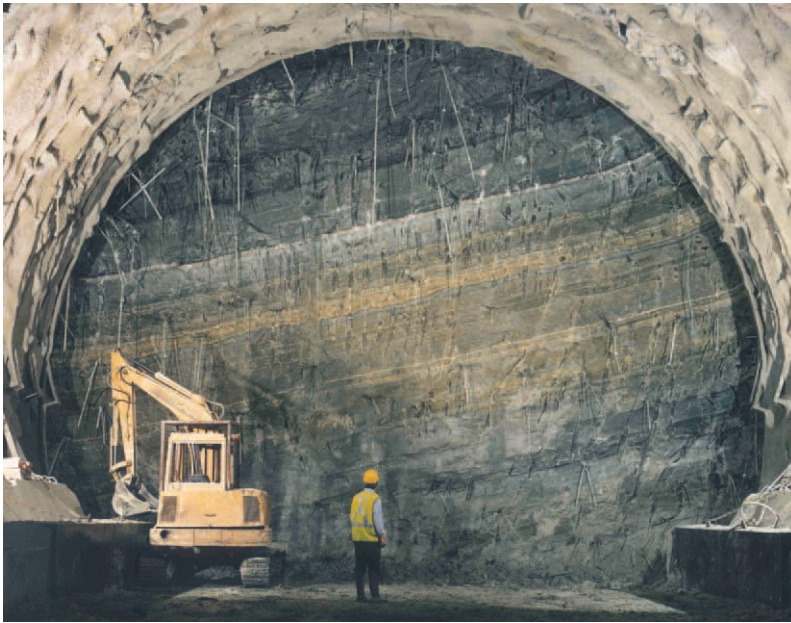
Fig. 23 TGV Méditerranée, Tartaignille tunnel: View of the face reinforced with fibre-glass structural elements.
