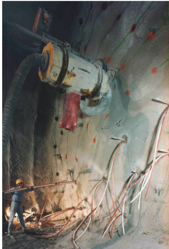
Fig. 15 Caserta to Foggia rail line, San Vitale tunnel: reinforcing the advance core using tubular fibre-glass elements.
