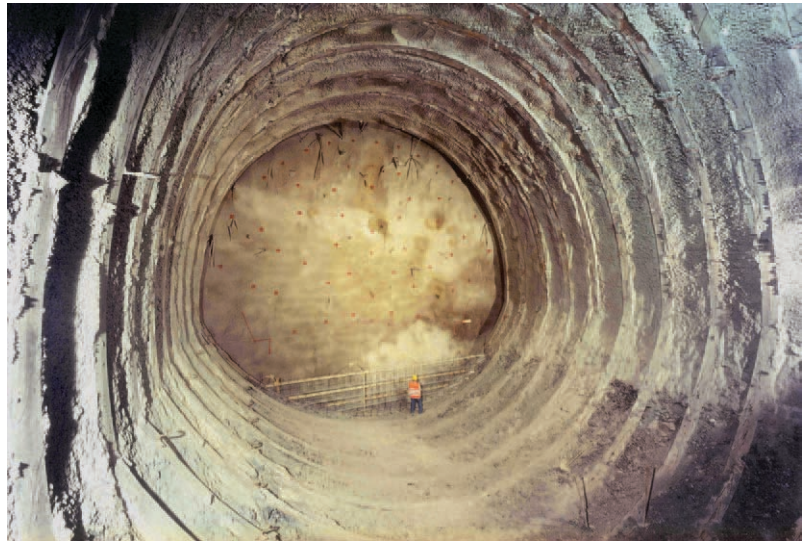
Fig. 25 Bologna to Florence High Speed Rail Line, Raticosa Tunnel: view before casting the invert near the face.
