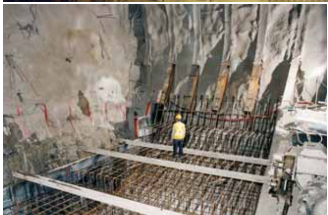
Figure 15. Invert cast near the excavation face - Raticosa Tunnel (Diam. = 13.90 m, Ground: scaly clays, Coverage: 500 m) and Tartaguille Tunnel (Diam. = 15.30 m, Ground: swelling clays, Max. overage: 150 m).
