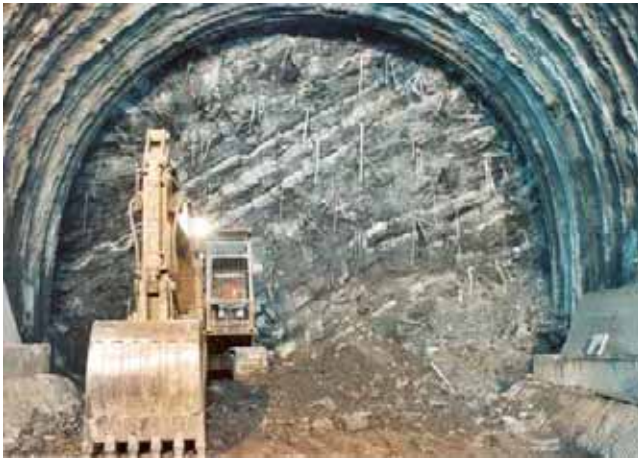
Figure 23. Monte Bibele Tunnel, the core-face reinforced with fibre-glass structural elements (ground: Monghidoro flysh).
