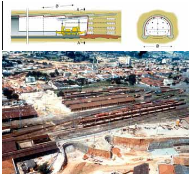
Figure 2. Protection of the core-face with full-section horizontal jet-grouting - Road underpass of the Campinas Railway yard (Diameter = 14.9 m, Ground: sandy, Coverage 2 - 4 m)
