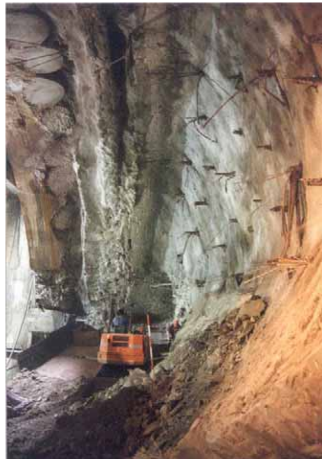
Figure 13. Excavation face shaped with a concave profile – tunnel of Baldo degli Ubaldi Station - (Diam. = 21.5 m, Ground: clay, Coverage: 15 - 18 m)
