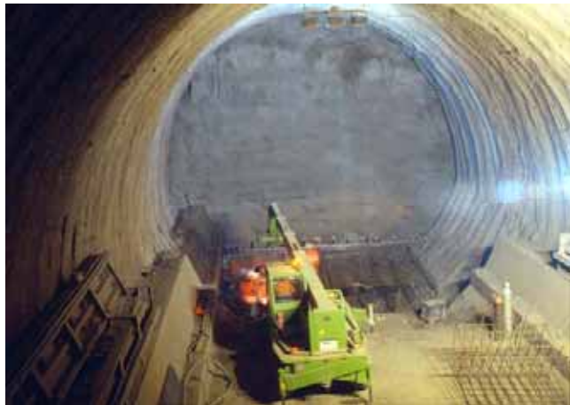
Fig. 14. Moving the casting of the invert away from the excavation face means increasing the extrusion surface
