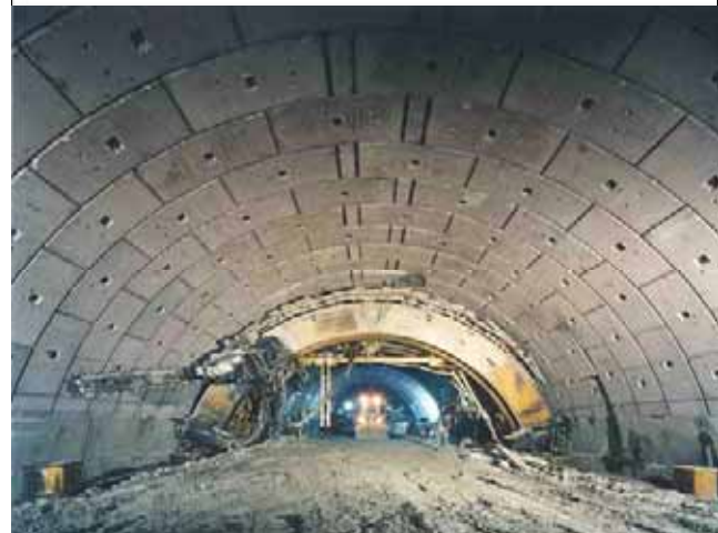
Figure 12. Mechanical pre-cutting – Baldo degli Ubaldi Station - (Diam. = 21.5 m, Ground: clay, Coverage: 15 - 18 m)
