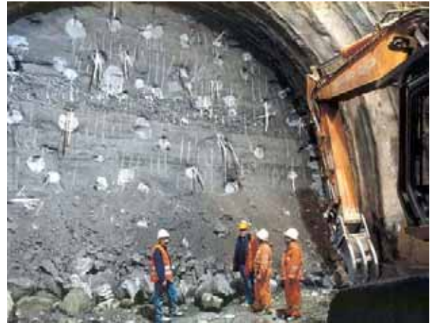
Figura 24. Firenzuola Tunnel, the core-face consolidated with reinforced micro-jet-grouting (ground: clayey sands with pebbly intercalations).
