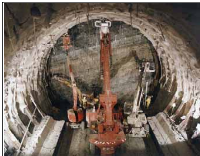
Figure 3. "Tartaignuille" tunnel (France), (Diam. = 15.30 m, Ground: swelling clay, Max. coverage: 150 m.
