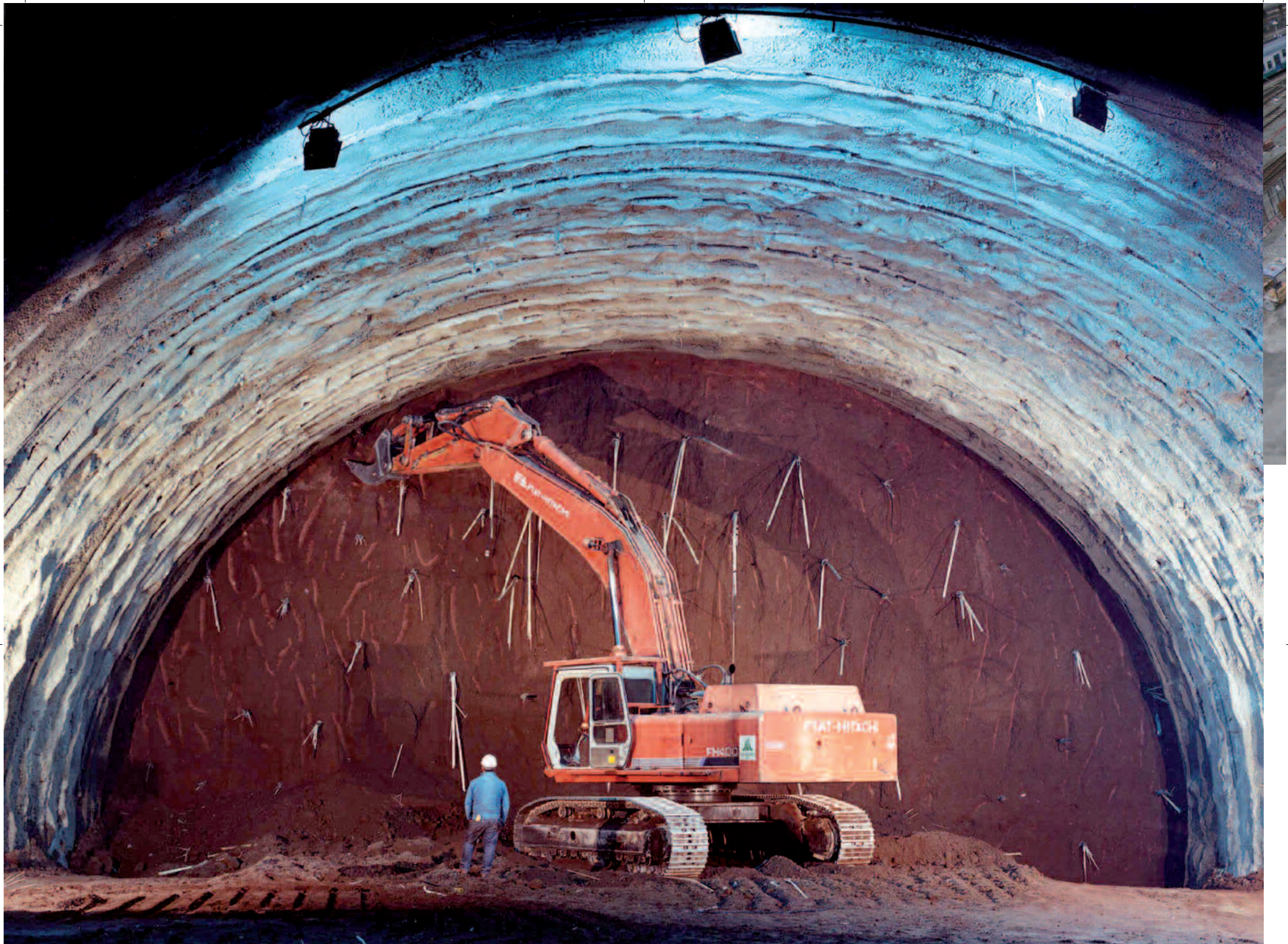
APPIA ANTICA TUNNEL ROME MOTORWAY RING ROAD Ø = 20.65 M. GROUND: GRANULAR PYROCLASTITES MAX. OVERBURDEN: ~ 4 M.
