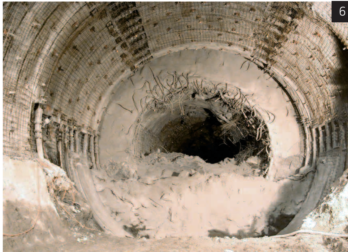
6. YIELDING SUPPORT SYSTEM WITH TH STEEL SETS AT THE GOTTHARD BASE TUNNEL (COURTESY OF ALPTRANSIT GOTTHARD AG)
