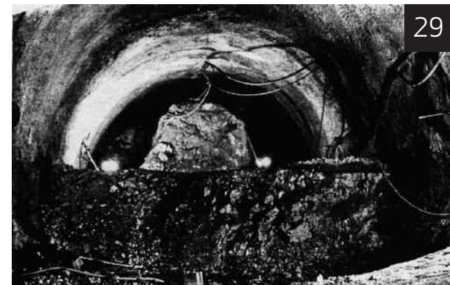
29. RABCEWICZ'S STABILIZATION OF THE TOP HEADING FACE BY USING A "NOSE" OF GROUND
