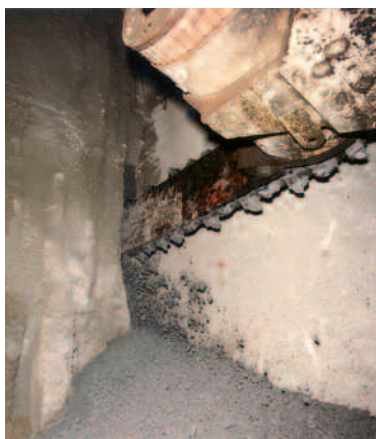
MECHANICAL PRECUTTING
