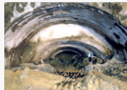
Tasso tunnel: collapse of the cavity (c)
