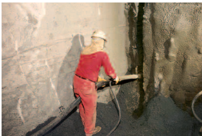
DETAIL OF MECHANICAL PRECUT AND FILLING THE PRECUT WITH SHOTCRETE
