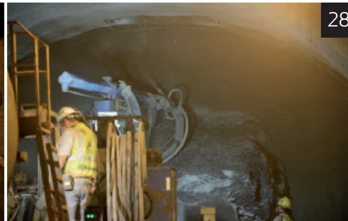
27. DEVIL'S SLIDE TUNNEL PROJECT, CALIFORNIA, USA. TOP HEADING AND BENCH EXCAVATION
