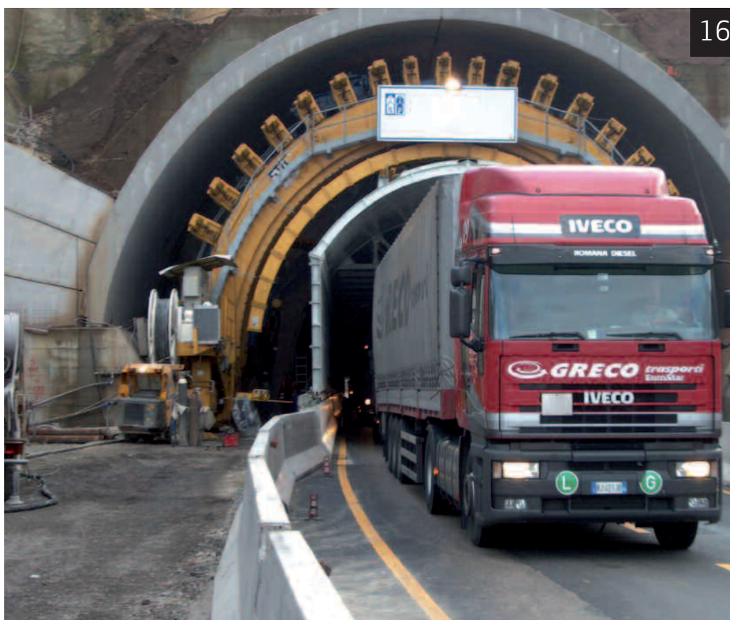
15. PLACING AN ARCH OF THE PREFABRICATED SEGMENT LINING
