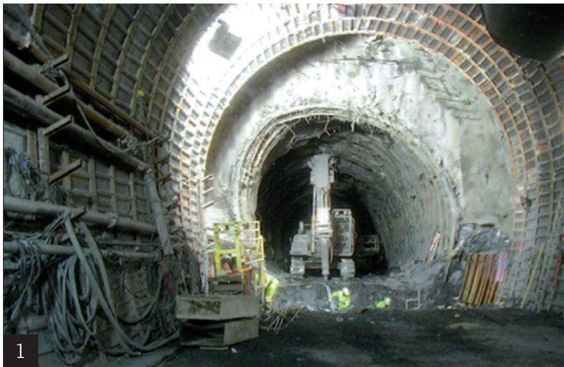
1. "SQUEEZING ROCK" REDUCES THE TUNNEL CROSS SECTION AS WELL EVIDENCED IN THE SAINT MARTIN LA PORTE ACCESS ADIT ALONG THE LYON-TURIN BASE TUNNEL
