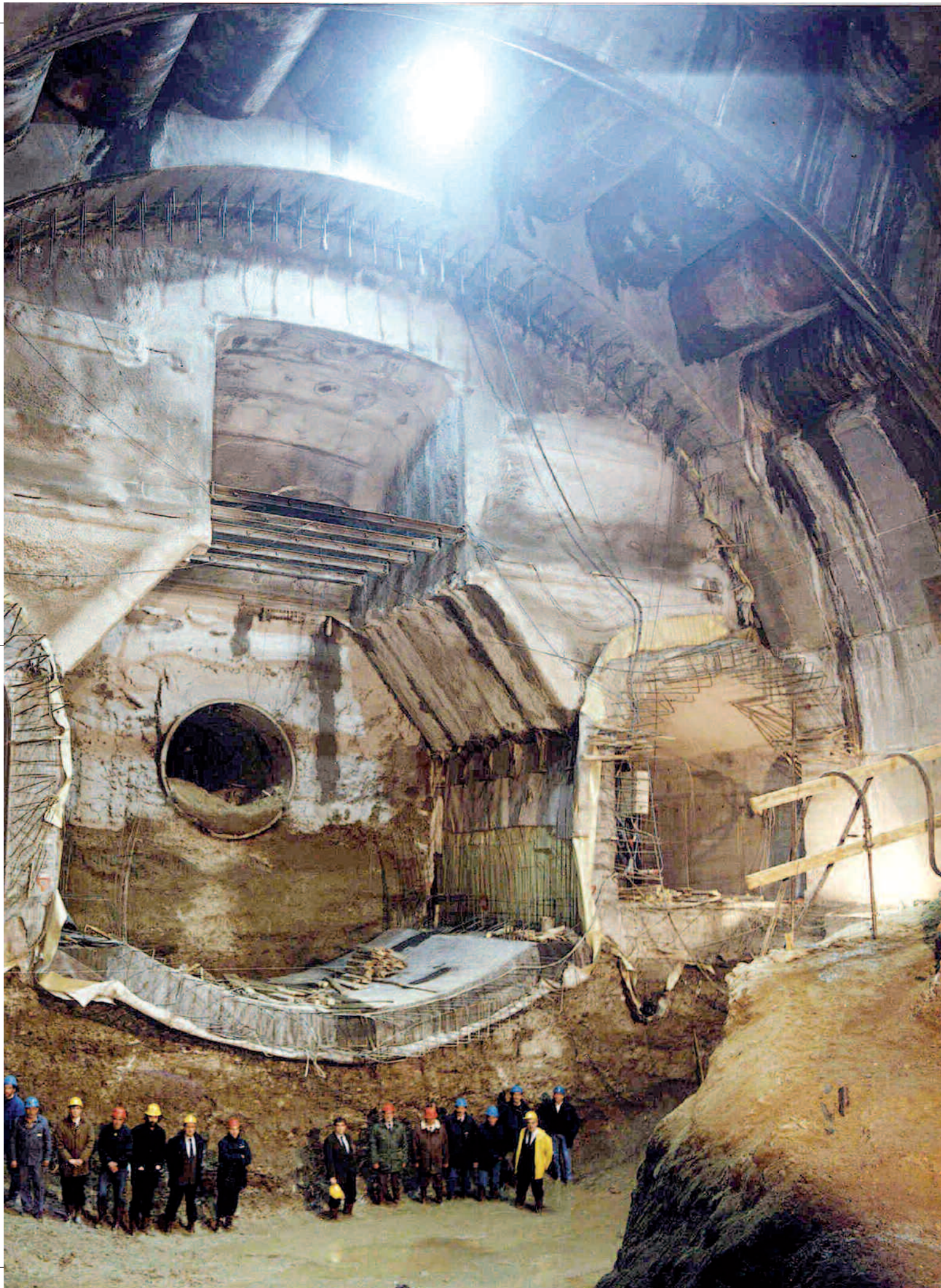
VIEW OF VENEZIA STATION AFTER COMPLETION OF EXCAVATION UNDER THE PROTECTION OF THE CELLULAR ARCH CROWN THE MILAN URBAN LINK RAILWAY LINE
