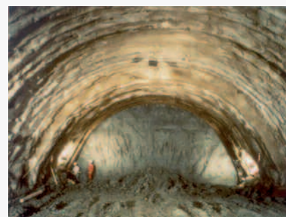
Tasso tunnel: half face advance (a)
