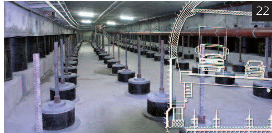
22. CHIENBERG ROAD TUNNEL AFTER COMPLETION: "MODULAR YIELDING SUPPORT"
